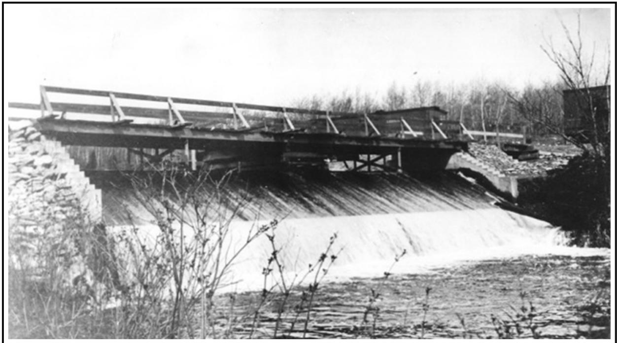
Beaplant Dam No. 2 (Plant No. 3); (Dam No. 3, Plant 4 No Photo)
