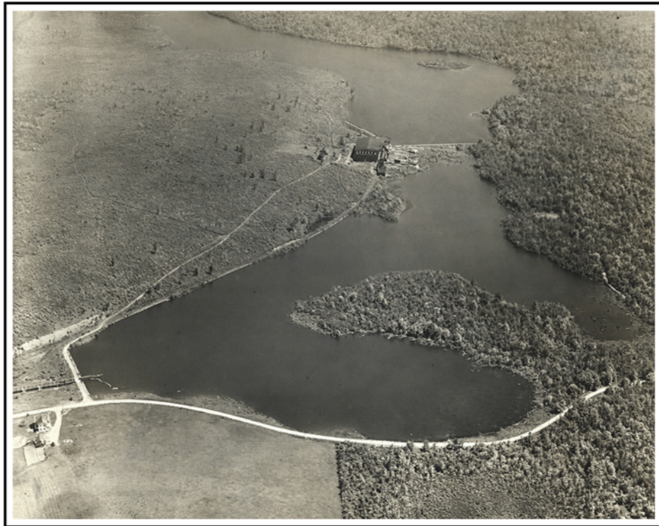
Meadow Run Lakes – Dam No. 4 (No Plant) and Dam No. 5 (Plant 6)
