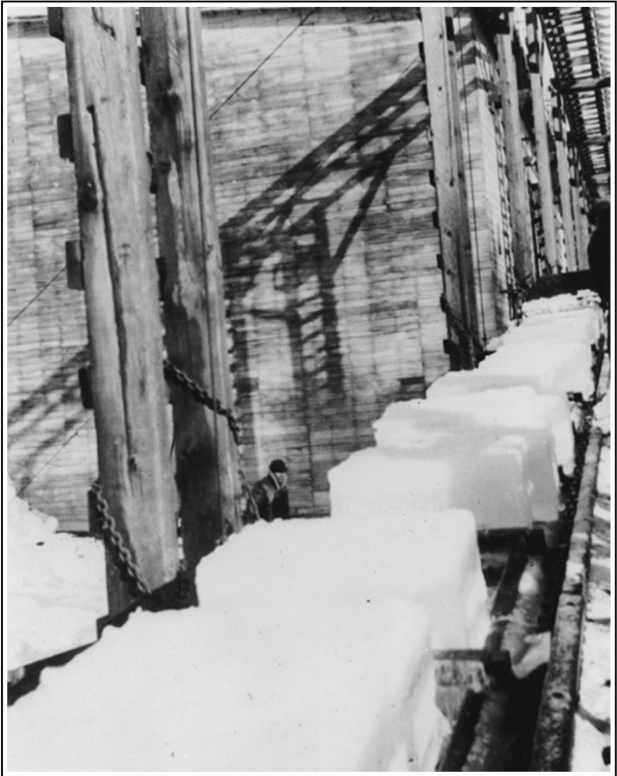
Ice Cakes Carried up Conveyor to Ice House
